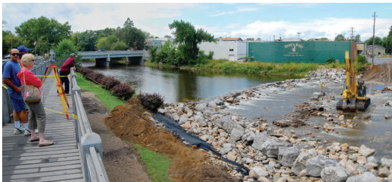
Construction on Chesaning weirs. Photo by Gail Krantzberg.
